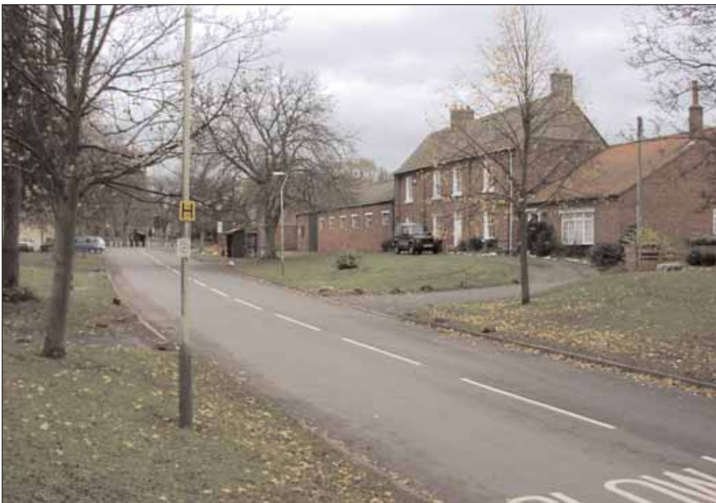
View towards Grade II listed Manor Farm, The Green
